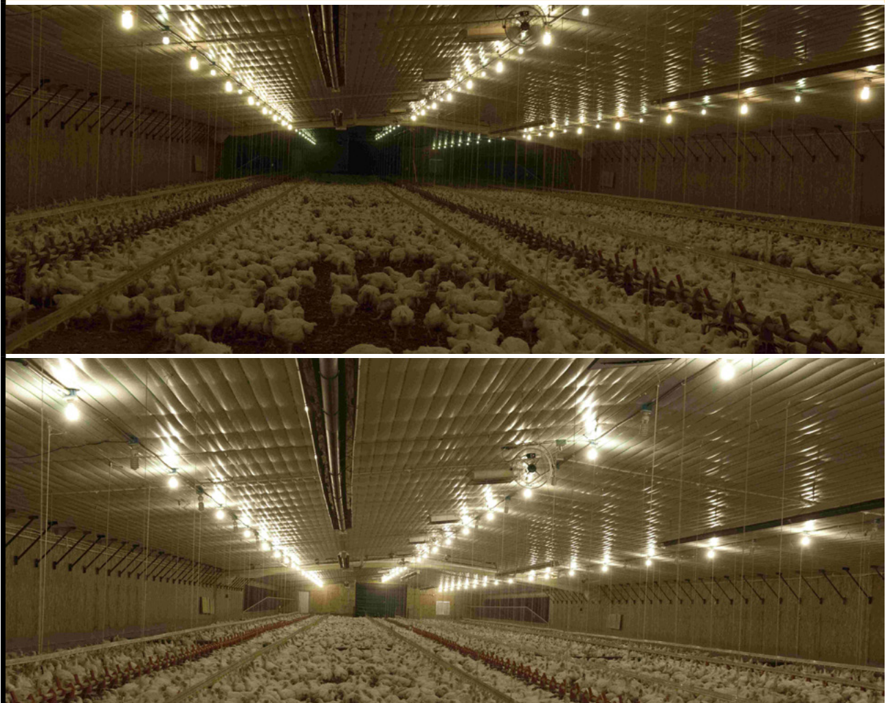
Figure 6.30 Example of 10 lux / 1 fc (top) and 30 lux / 3 fc (bottom) light intensity.
