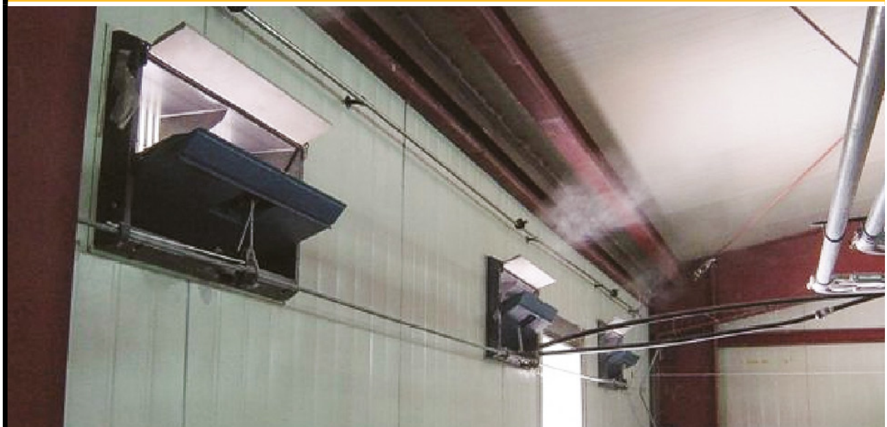
Figure 6.25 Example fogging system for a cross-ventilated house.
