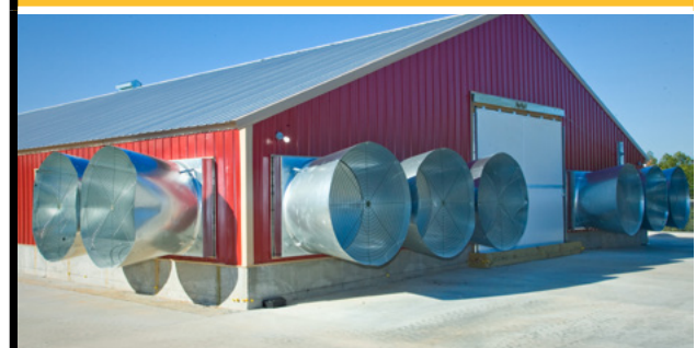
Figure 6.17 Example of a typical tunnel-ventilated house.
