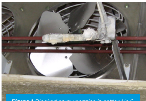
Figure 1 Blocked spray nozzles in setter No.6
