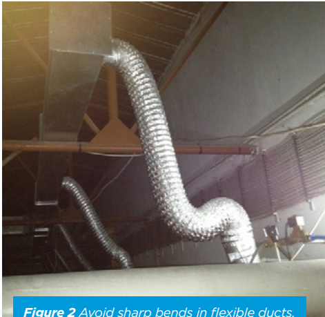
Figure 2 Avoid sharp bends in flexible ducts.
