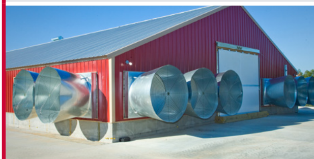
Figure 6.17 Example of a typical tunnel-ventilated house.
