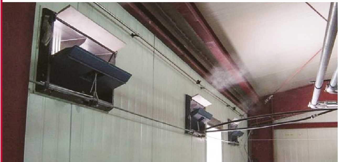
Figure 6.25 Example fogging system for a cross-ventilated house.
