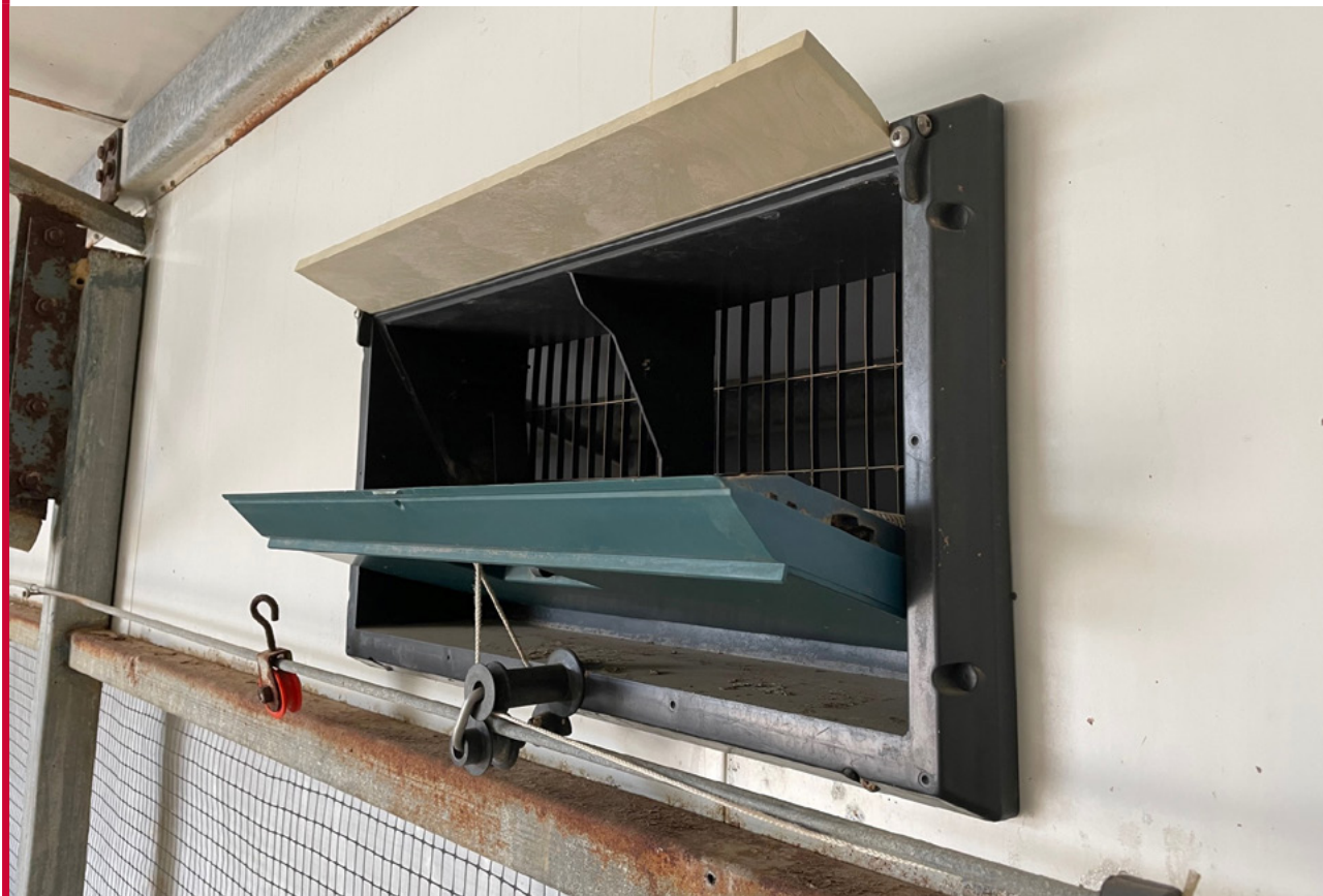
Figure 6.10 Example of a good-quality air inlet.
